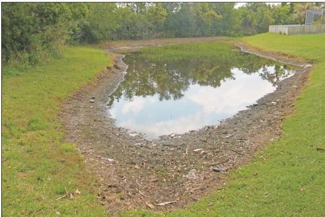
This pond is subject to erosion all the way around without perimeter plants.
