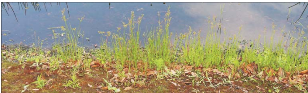
Photo below shows lack of plants and bank sod leading to pond erosion. Photo above shows plants springing up on their own that help stop erosion in the critical area where pond slopes meet pond banks. Photo at right shows erosion starting at hard-to-see, black plastic pipe within the circle.
