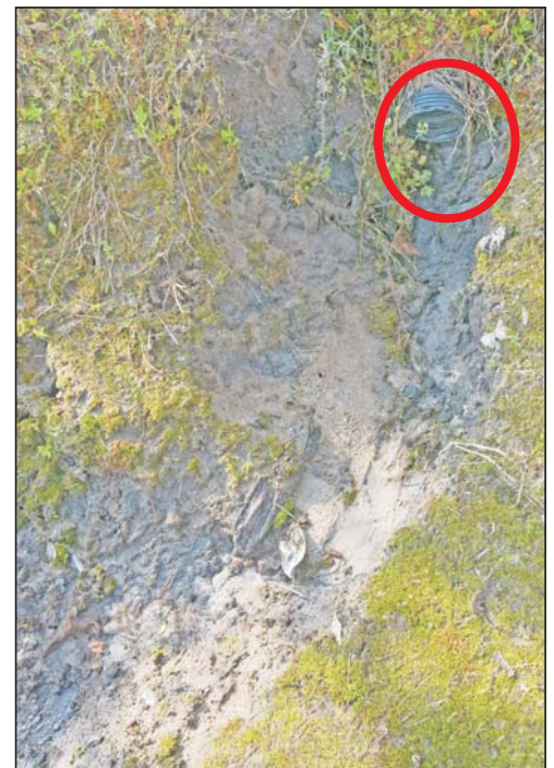
Photo below shows lack of plants and bank sod leading to pond erosion. Photo above shows plants springing up on their own that help stop erosion in the critical area where pond slopes meet pond banks. Photo at right shows erosion starting at hard-to-see, black plastic pipe within the circle.
