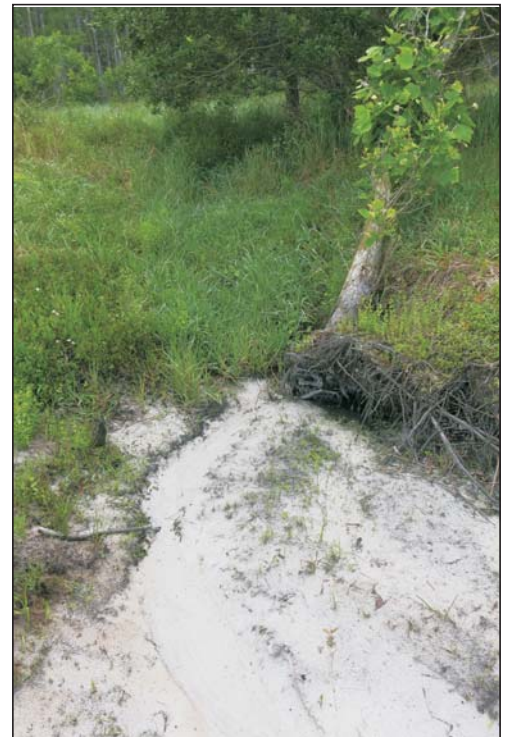
Photo at right shows increasing erosion that downed a tree on Pond 13 and blocks vendors from accessing the back side of the pond. Above, circle shows location of piping that carries water from Pond 13 in Castleway under Ballantrae Blvd. and into Pond 12 in Cunningham.
